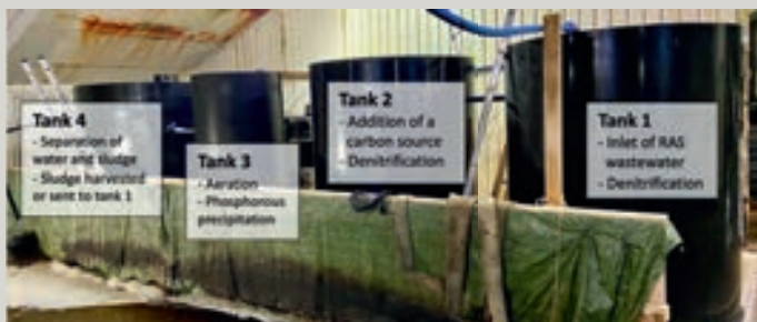
Figure 1. A small-scale active sludge system. In tank 1 wastewater from RAS is added and denitrification begins. In tank 2 a carbon source such as sludge or methanol is added to increase the efficiency of denitrification. The water and sludge are then let to tank 3 where phosphorous is precipitated and aeration is added to release N_2 to the air. Finally, in tank 4, water and sludge are separated, and the sludge is harvested or returned to tank 1. The water is then discarded with much lower content of nitrogenous and phosphorous waste.
